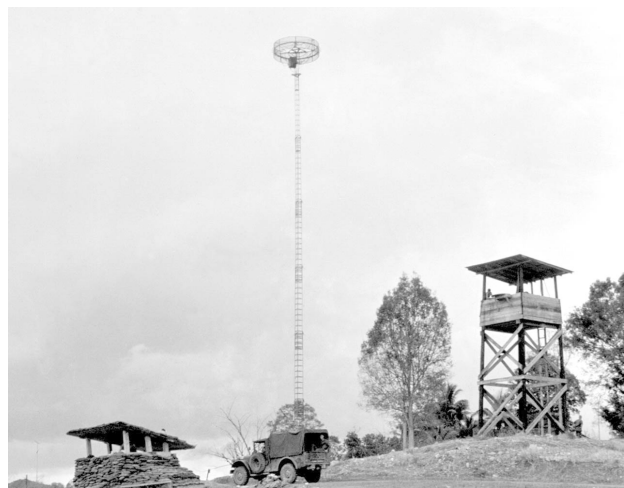
FIGURE 1. The Camp Sentinel Radar-II was first installed and operated in Lai Khe, Vietnam, in 1968. The system was situated on the perimeter of the U.S. Army camp, with the radar antenna mounted on top of the tower. The remainder of the radar system was located in a bunker behind the hill in this picture, where the machine-gun tower was located.
