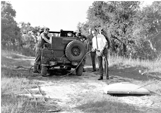
FIGURE 2. Field operation of the Geodar ground-penetrating radar system. Initial testing of this system consisted of dragging the antenna over a known test area to detect tunnel-like voids under the surface. The antenna was connected to the radar equipment in the jeep by a cable.
