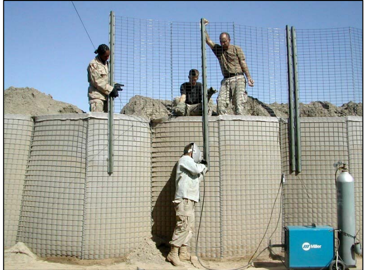
For maximum protection along Camp Griffin's north perimeter, the DEMONS erected a 375 foot long, homemade, experimental, anti-RPG fence on top of the Hesco barrier wall.
