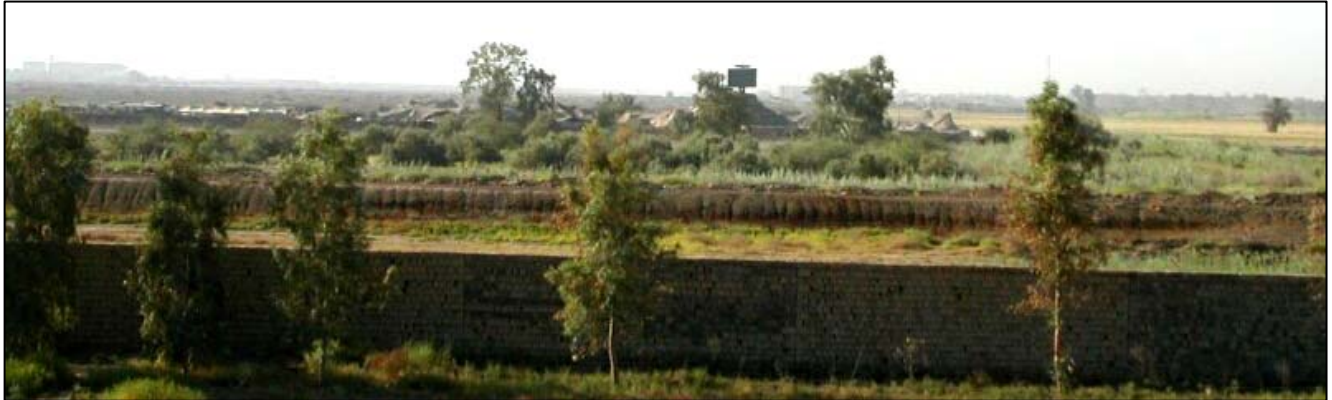
A look at Camp Griffin from the top of a house outside the Airport's north wall. The mission outside the wall was to assess Camp Griffin's defenses and concealment from the "enemy's" perspective. Twelve days later the enemy attacked Camp Griffin with mortar fire. The tower and terminal are visible in the far left background of the picture.
