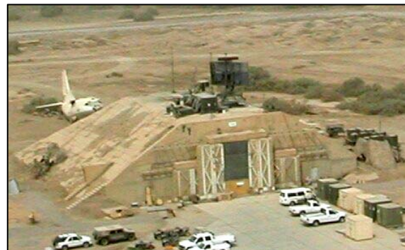
Radar "B" set up on top HAS 4, Combat Search and Rescue squadron set up inside the HAS.
