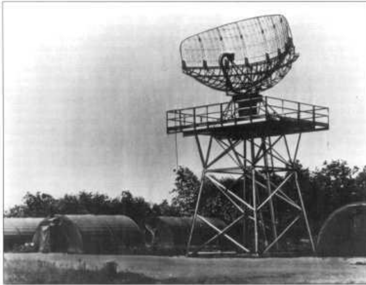
AN/CPS-5 radar; the basic unit of the Lashup system (Photograph courtesy Air Force History Support Office)
