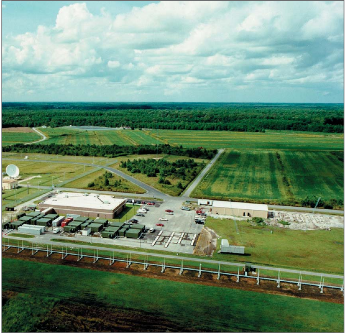
Consolidated Operations Control Center at Virginia Receive Site
