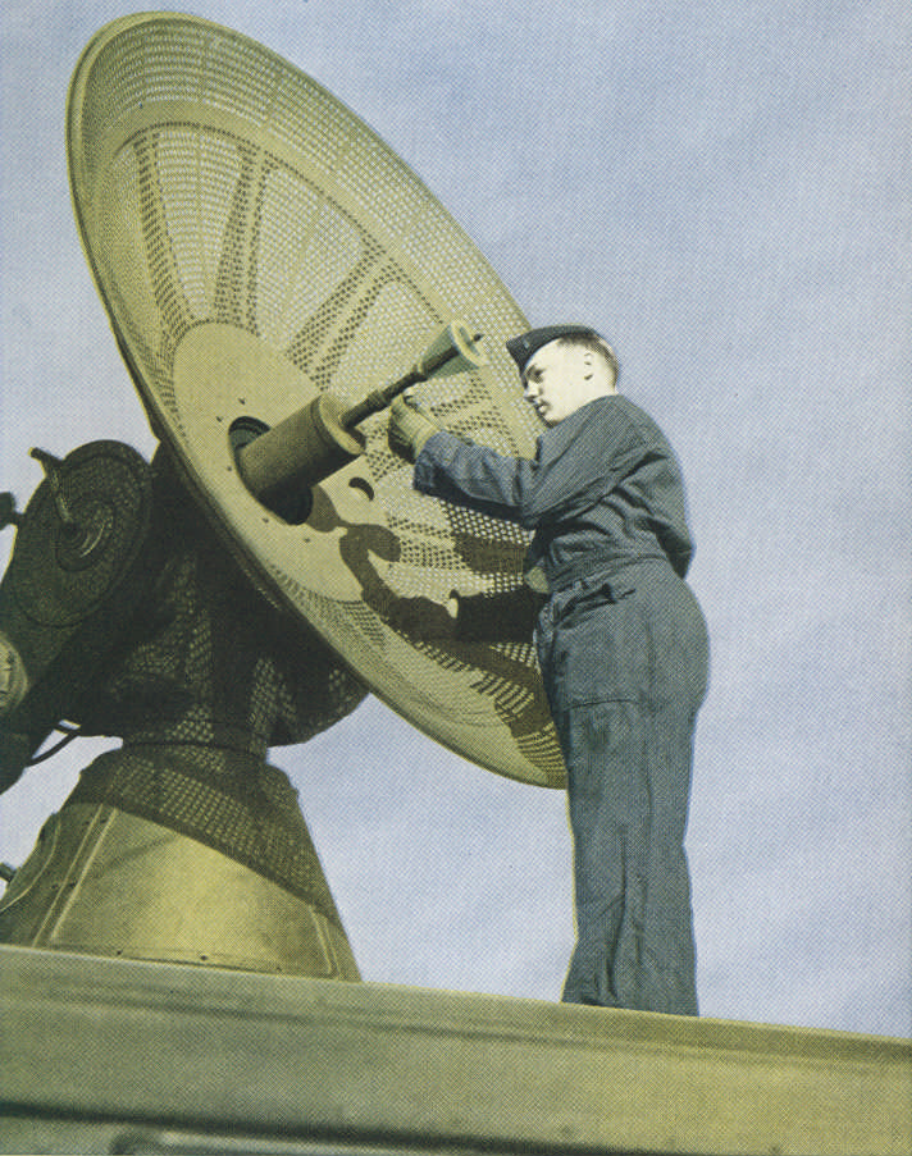
Signal Corps officer attaching the plastic-enclosed radar antenna to the spinner motor.
