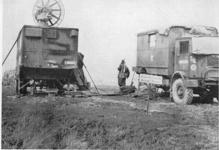
Recording van on right made records of radar operations for the study of anti-aircraft research groups.
