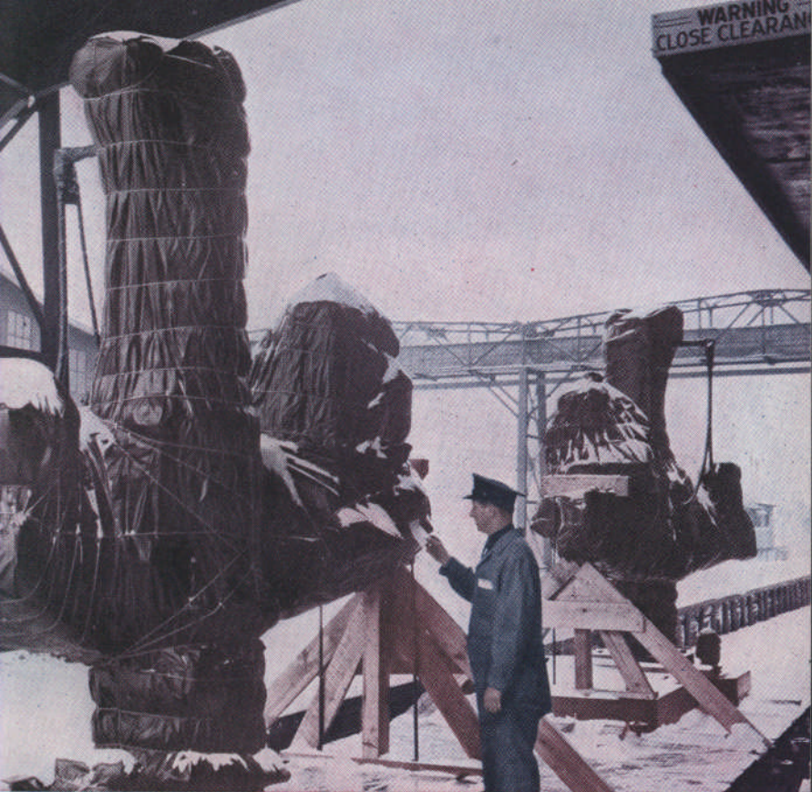
Radar-making machine tools begin to arrive at the Dodge Plant. These are radial drills in their shipping wrappers.
