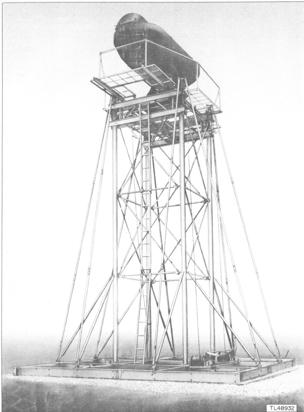
Figure 2-34. Tower completely erected.
